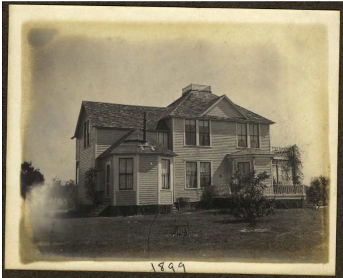
The kitchen extension and bay window on first floor have been added. The 1899 date is possibly correct.
