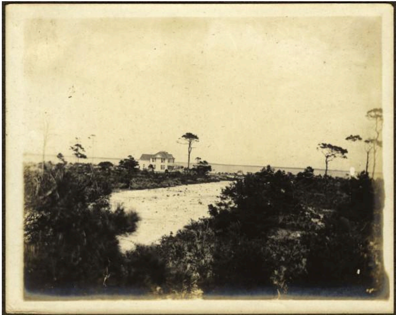
Green Gables soon after construction. This photo was taken from the west, perhaps about at the railroad tracks. The newspaper commented that Mr. Wells built his house way north of town. The light area is sand.
