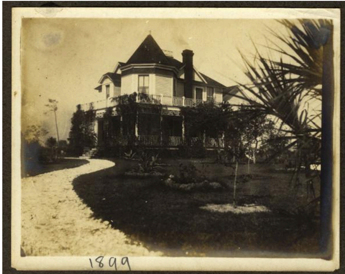
Here you can see the addition of the turret, the extension of the second floor of the kitchen wing, and the addition of an entrance to the second floor porch from the front of the house. The original entrance to the second floor porch is a door just to the right of the chimney in this photo. That door still exists and opens off the hall that leads to the turret room. The 1899 date is incorrect.
