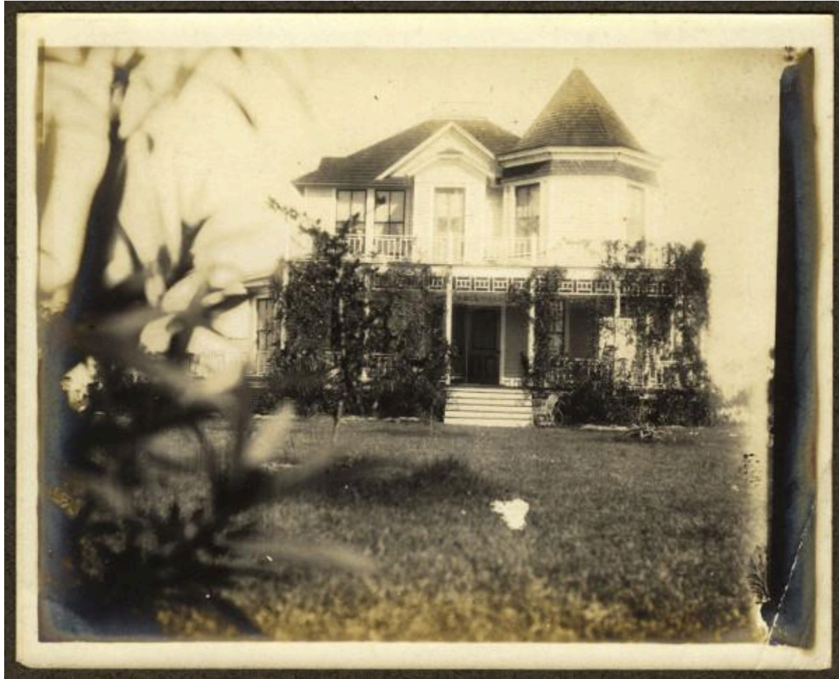
Another view of the south elevation prior to addition of the second floor bay window.
