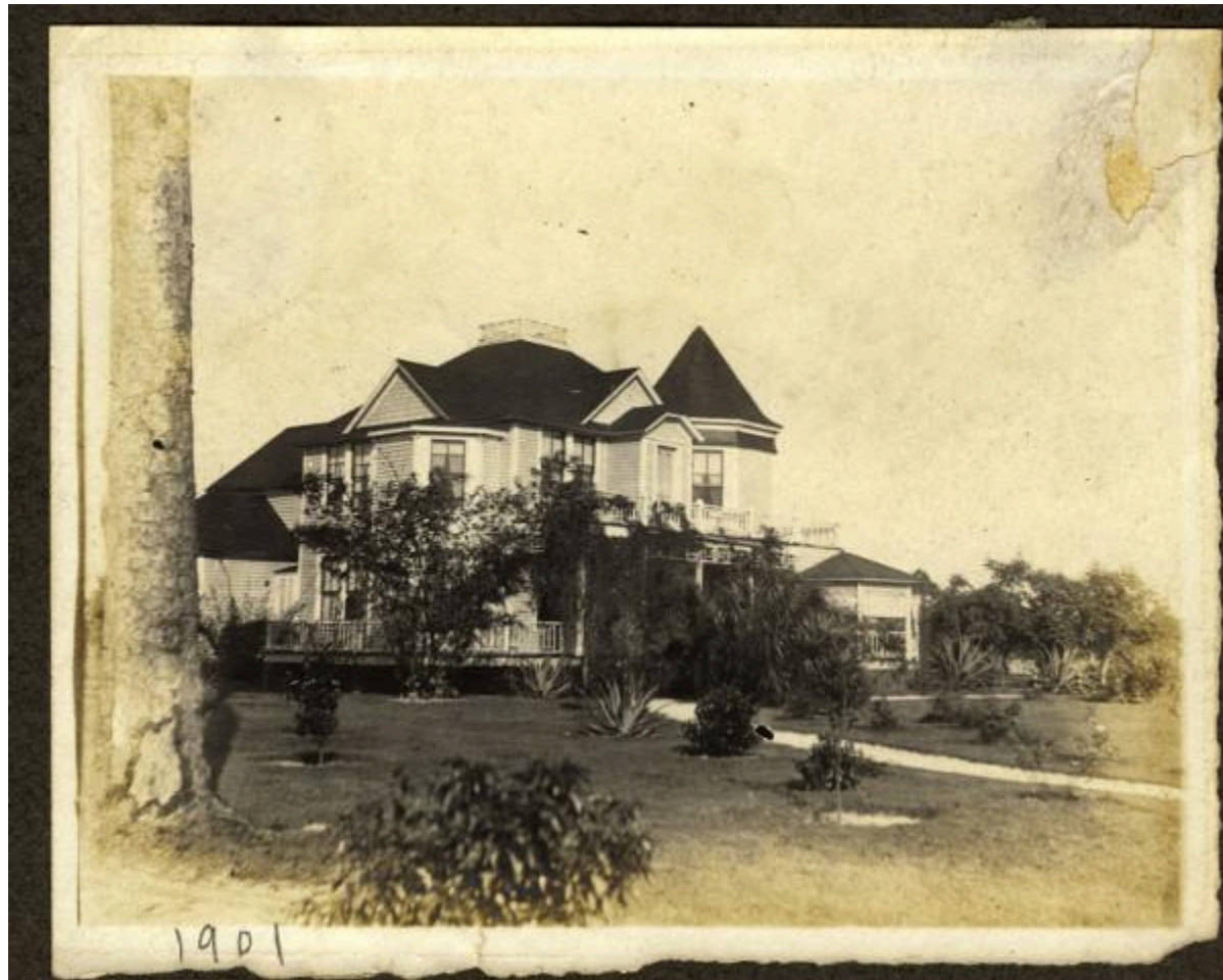
And here is the configuration that we want to restore with the addition of the second floor bay window. The 1901 date is incorrect.
